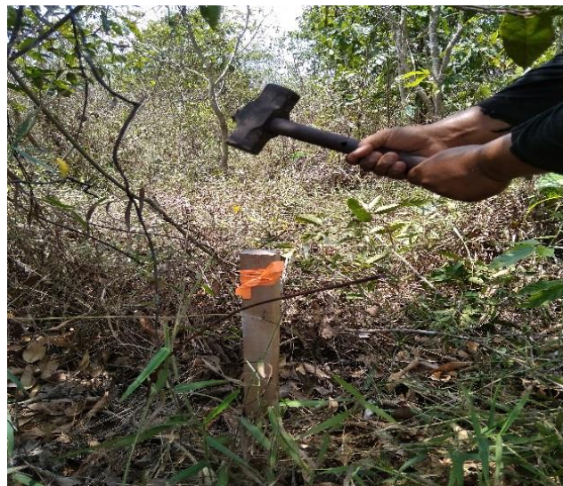
Gambar. 2 Pre-Marking titik GCP
